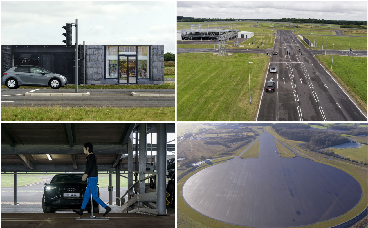
Figure 4-2: ASSURED CAV facilities in HORIBA-MIRA Proving Ground
